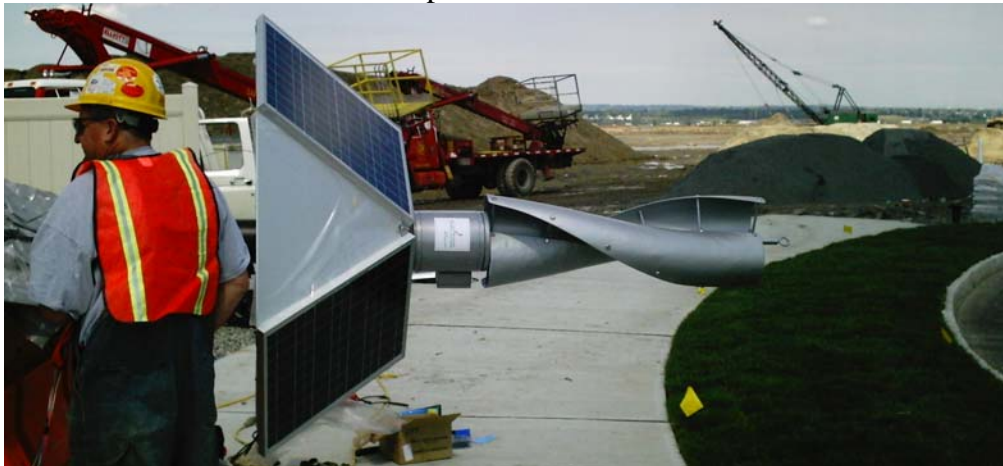
4. Mount Turbine On Pole on Top of Solar Umbrella
