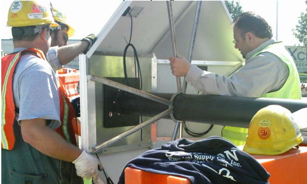
3. Assemble solar umbrella to pole top on ground
